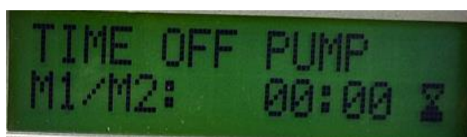
Fig.5. Main panel – lower end position
