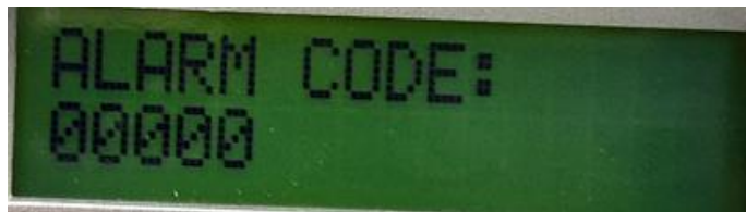
Fig.9. Alarm code panel
