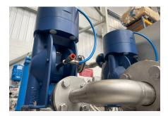
2x Tapflo Diaphragm Pumps with built-on Pulsation Dampeners.
