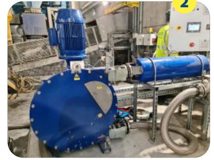
Phase three - commissioning, testing, and running the pump system
