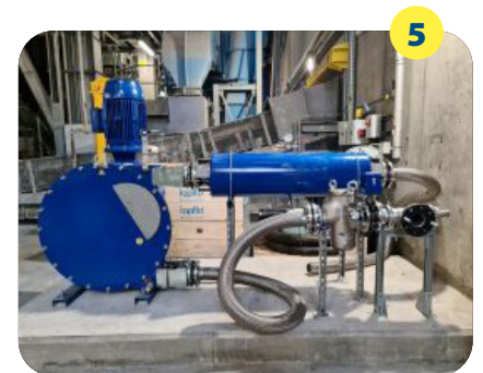
Phase one installation before panel and further supports
