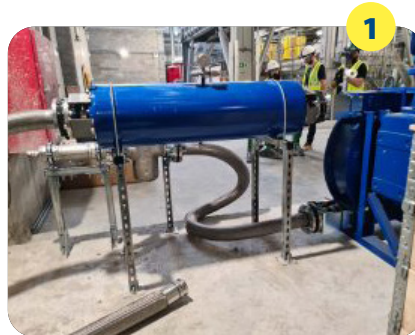
Pulsation dampener fitted to pump discharge during installation
